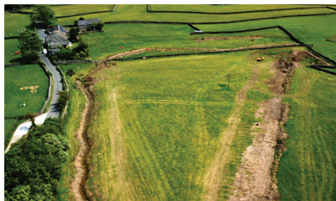
Above: Aerial view showing old culvert being filled on the right and a new meandering stream course on the left.
